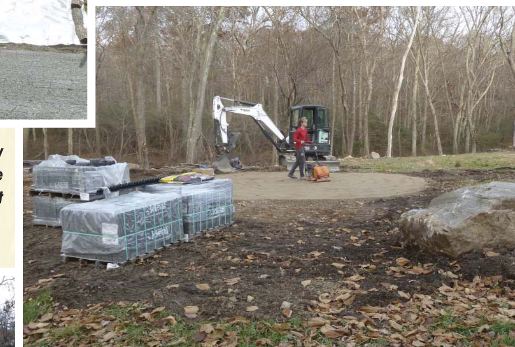
Left: VarsenScapes landscapers prep the site and install the paver circle
