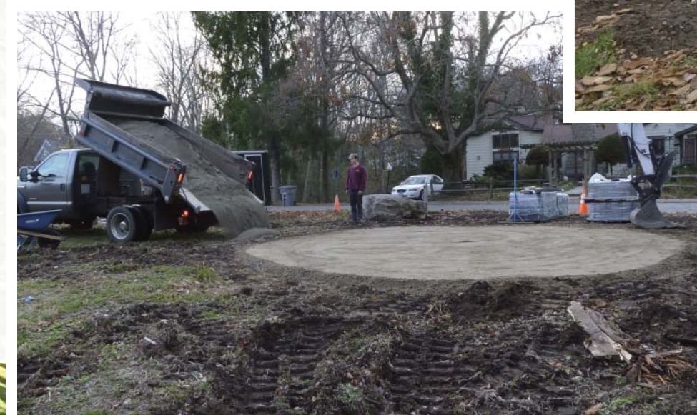
Left: VarsenScapes landscapers prep the site and install the paver circle
