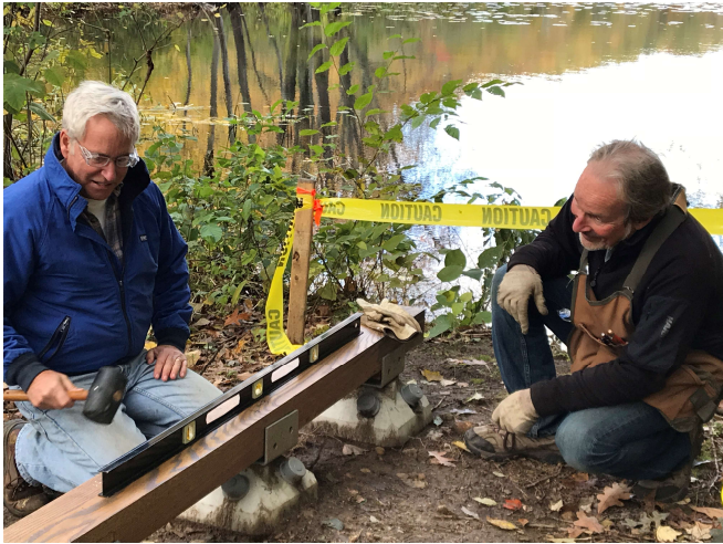
Greg Decker and Franz Edson leveling the foundation pins
